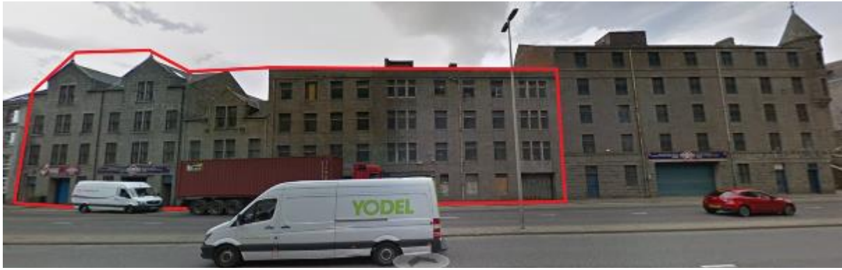
Photo 10: 12-14 Virginia Street and the unlisted 22-24 Virginia Street (outlined in red)
